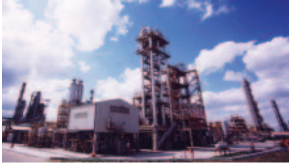
Right: MOGC's Moscow Refinery. Far right: Salym Crude Processing Facility
