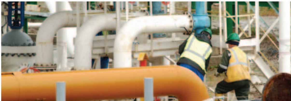
MAINTENANCE WORK IS ONGOING AT SALYM
