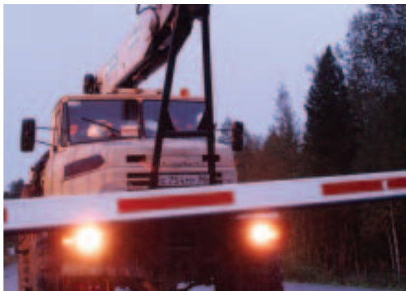
AT DUSK, WORK CONTINUES AT SALYM
