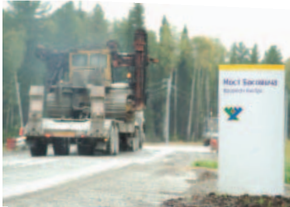
MOVING HEAVY EQUIPMENT AT SALYM
