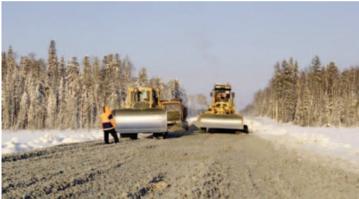
Above: Construction of the ComCor road at Salym
