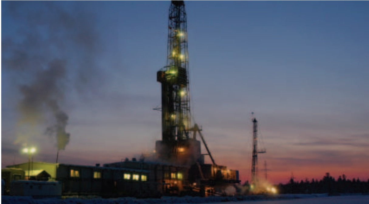
Above: Drilling continues around the clock at West Salym
