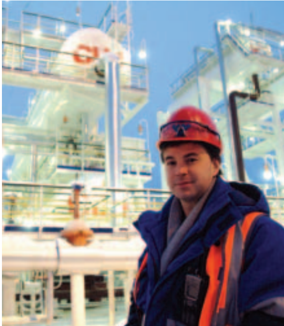
Above: Salym Crude Processing Facility
