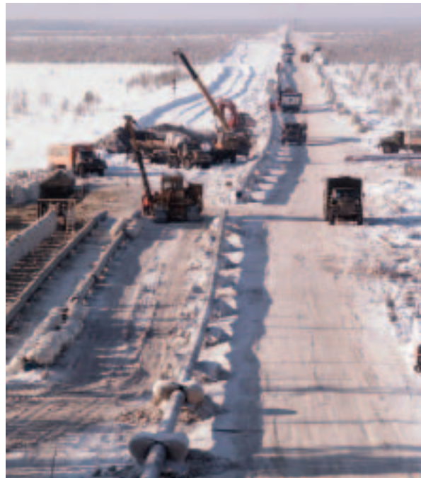
Above: Laying the 88km export pipeline at Salym
