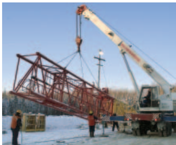
Above: Raising new drill rig.
