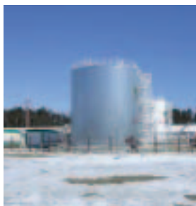
Below: Diesel and water tanks at Salym CPF.
