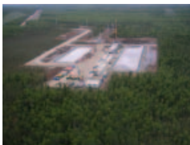
Right: Well pad 20 and Central Processing Facility.
